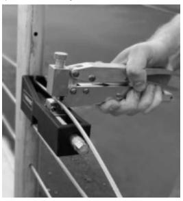
**4.** Connect the cable at the end post, without having to pull tension through the entire cable length, only from the pre-tensioner to the end post. After installing the cable at the end post, release the clamp and remove the pre-tensioner. Reset using the impact driver, and move on to the next cable, repeating the process.
