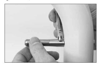
7. Pull the cable tightly along the side of the fitting and mark the cable 1-3/16" from the end of the fitting opposite the post. Mark and cut the cable on your mark.
